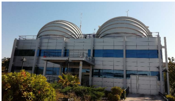
Figure 1: CEAM building with the 2 chambers on the roof
